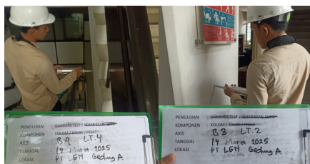
Figure 2. Hammer Test Inspection source: research data
