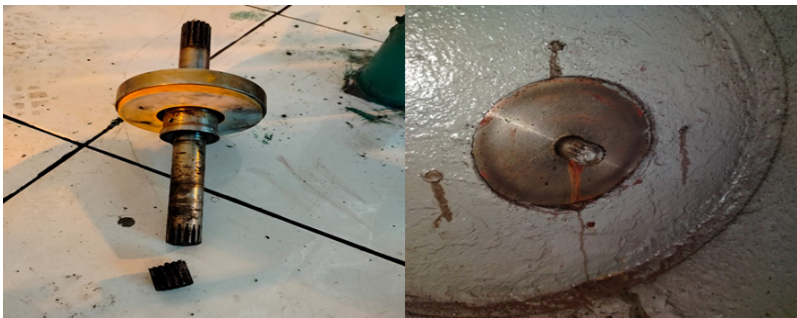
Figure 3. Shaft Fracture on HP Pump SWRO Date June 11, 2025 (Source: Private archive, 2025)
